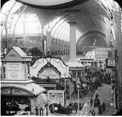
Electricity Building at Chicago World fair (1893), Brooklyn Museum
